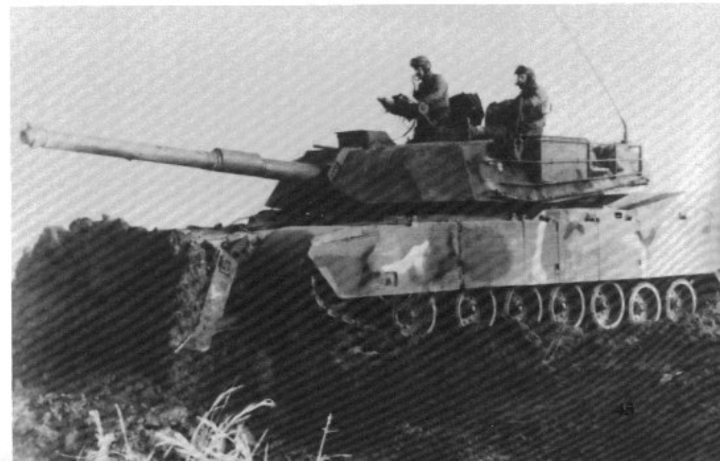
A dozer kit, modified from the M9 bulldozer used on the M60, was installed on the M1 at Fort Belvoir and tested at Fort Knox. Although successful, the tests indicated that a new dozer unit should be designed to take full advantage of the lower silhouette of the M1. (U.S. Army via Armor Magazine)
